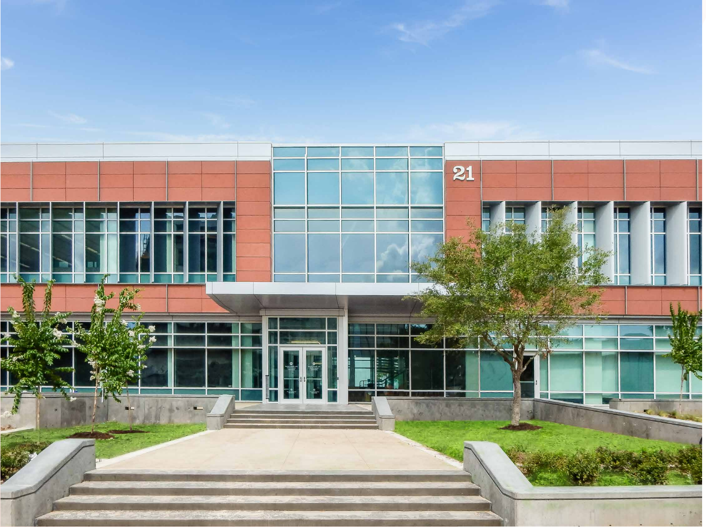
Red Sandstone Exterior Cladding NASA JSC Human Health and Performance Laboratory
